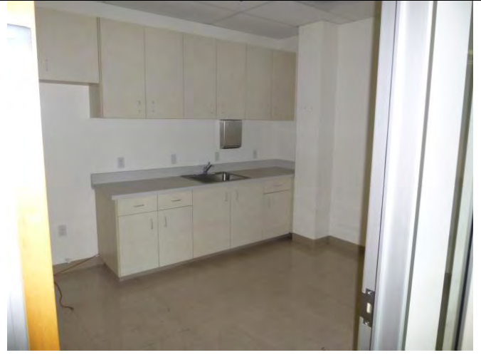
Typical Kitchen Space
