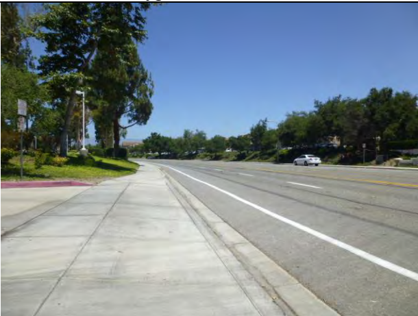
Northerly View Along Rancho Conejo Blvd.
