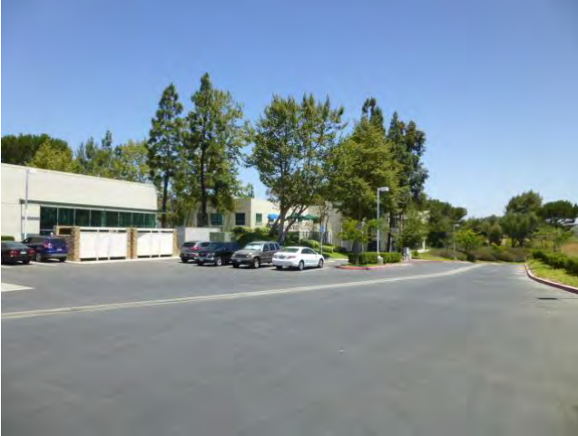
Rear of Building (1525 Rancho Conejo Blvd.)
