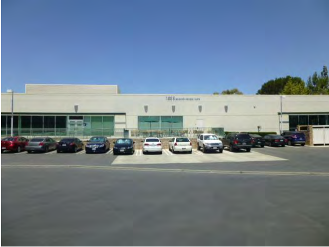
Rear of Building (1535 Rancho Conejo Blvd.)
