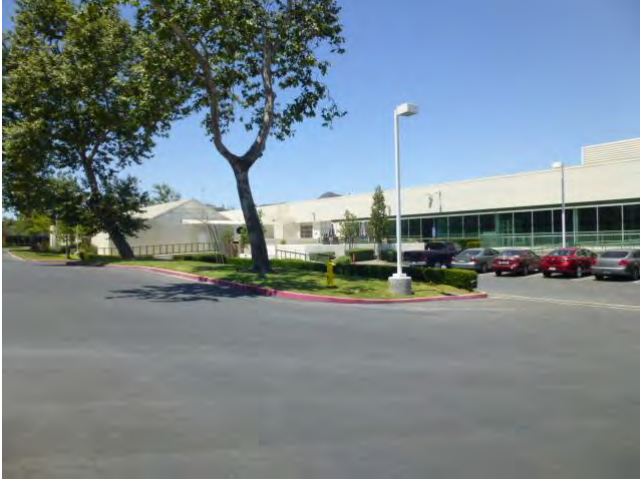
Driveway and Parking Behind both buildings
