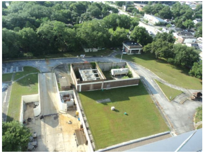
CHILLERS AND LOADING AREA
