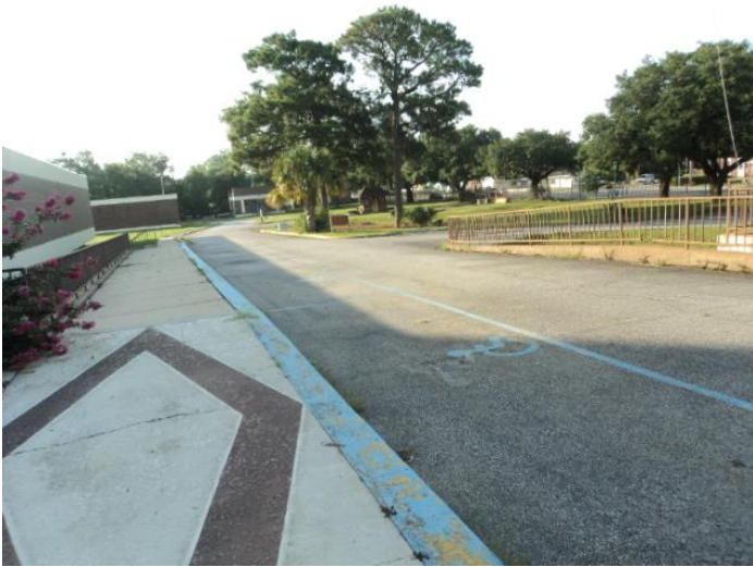
WEST SIDE ACCESS ROAD
