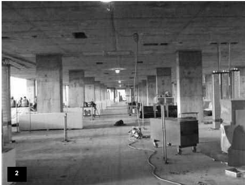
Tower Level T66 – View of the following in process items: domestic hot and cold water supply lines and vertical mechanical duct.
