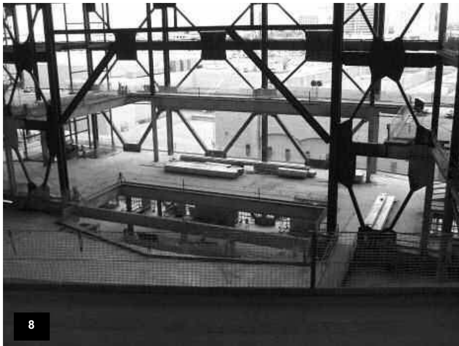
Podium – View looking south at the stage area in the theatre.
