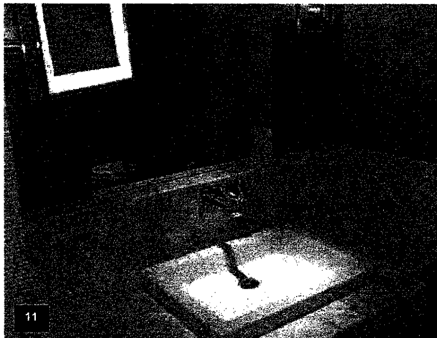
Tower Level T2 – View of a typical condominium bathroom completed including: vanity top, sink, mirrors, valance and faucet.
