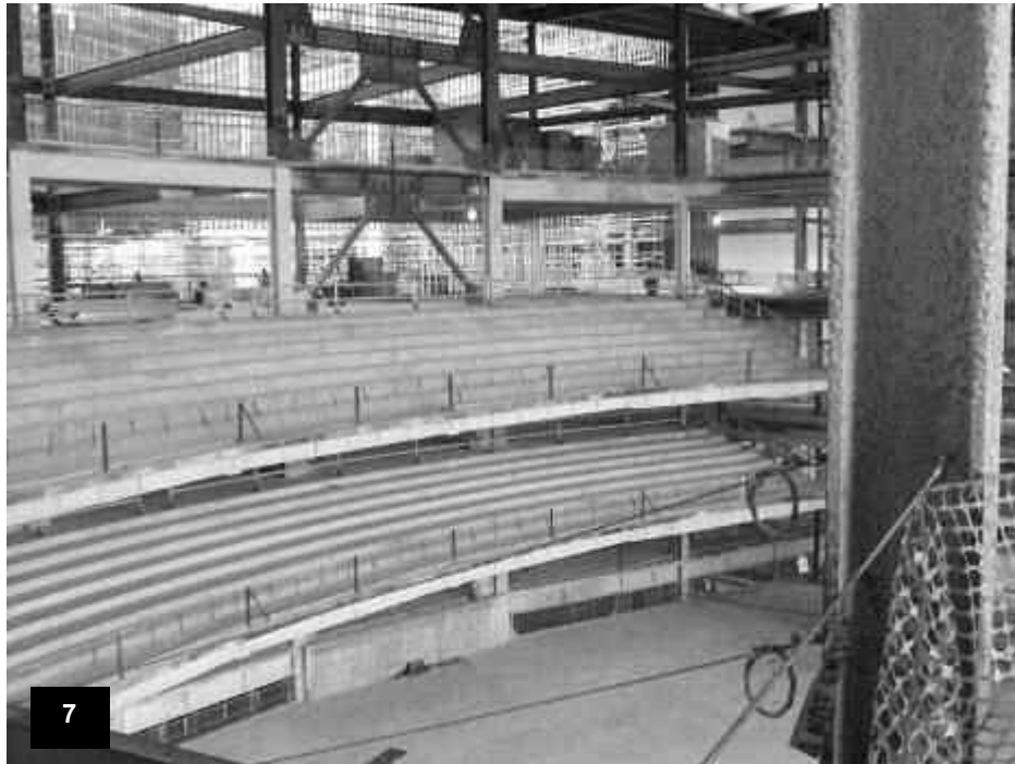
Podium – View of the completed concrete mezzanine seating in the theatre.
