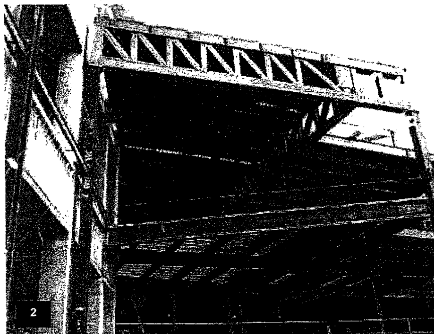
View of the Podium structural steel framing along Las Vegas Boulevard with the last truss scheduled for installation the second week in February.
