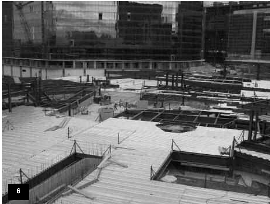
Podium Pool Deck – View of the structural steel framing and metal decking with pool, spa and escalator openings framed.
