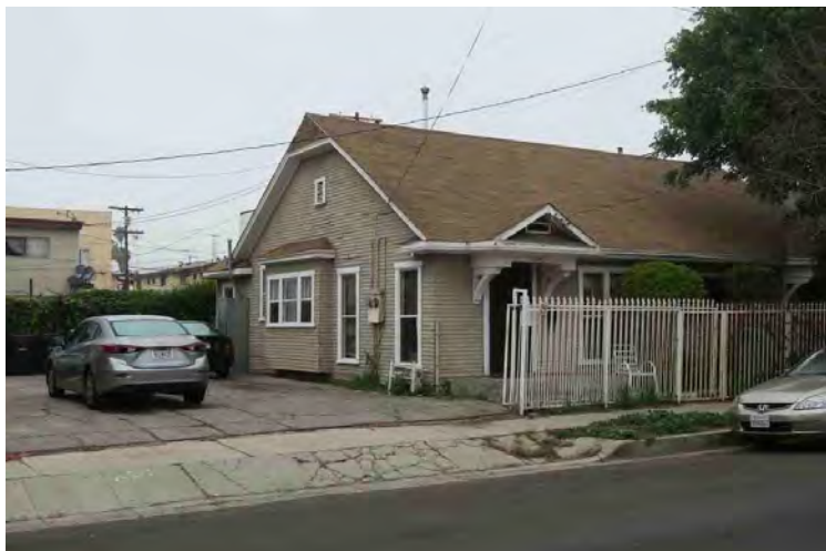
Lexington Avenue Building
