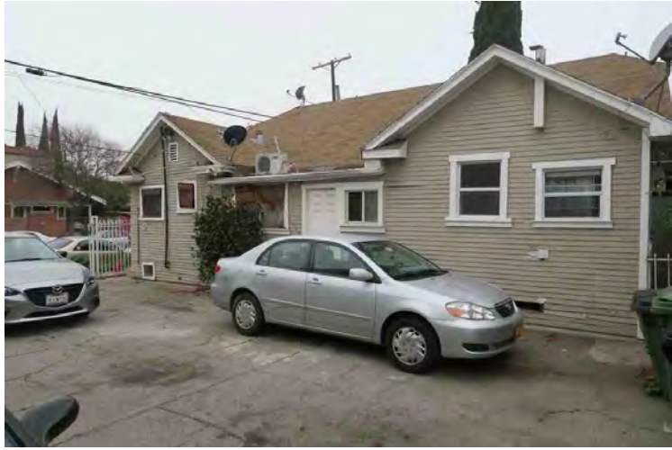
Rear of Gordon Street Building
