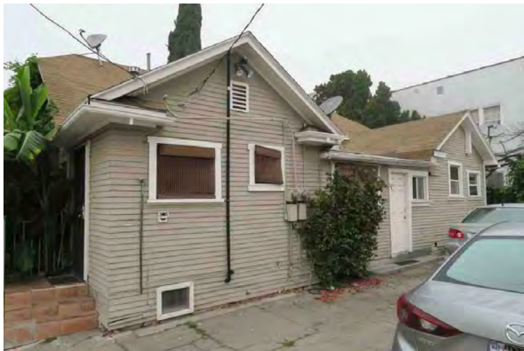
Rear of Gordon Street Building
