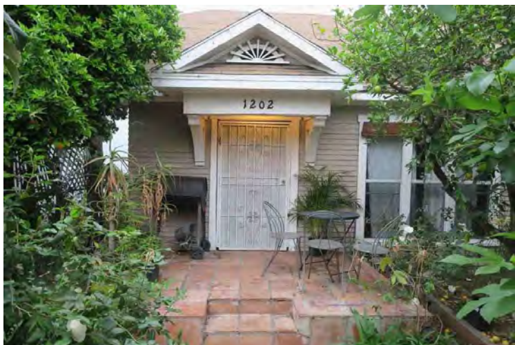
Front of 1202 Gordon Street
