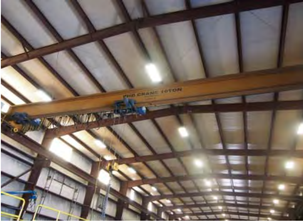
BRIDGE CRANES BUILDING 1
