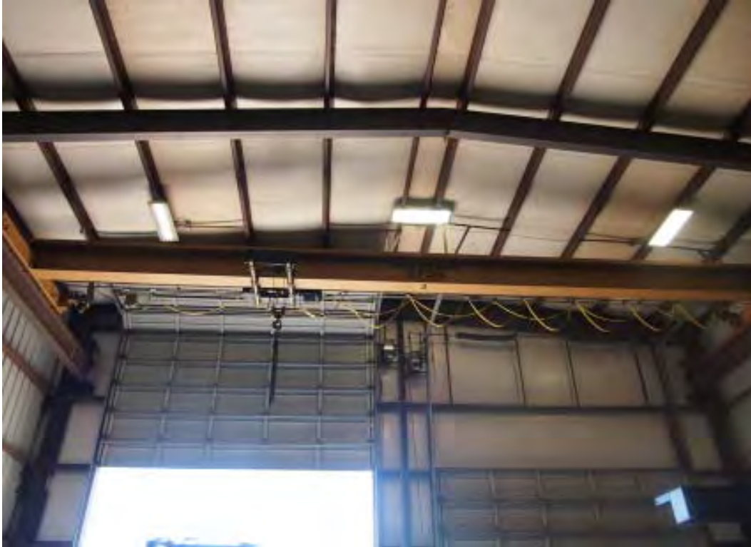
BRIDGE CRANES BUILDING 2
