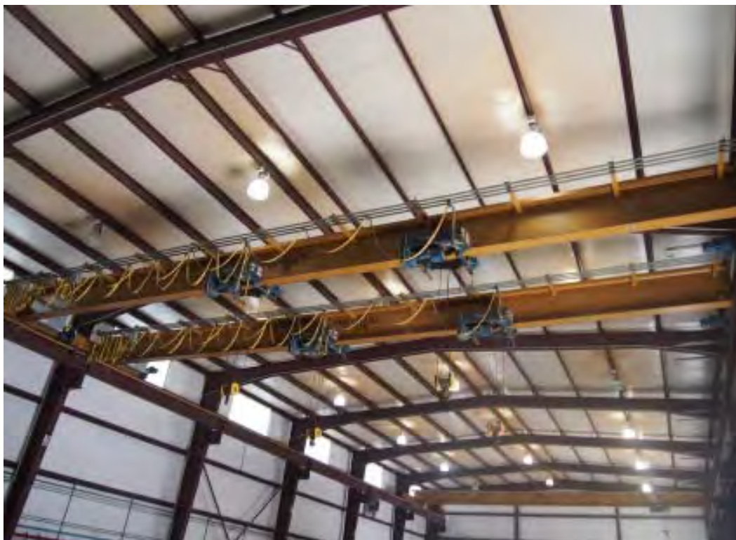
BRIDGE CRANES BULDING 4
