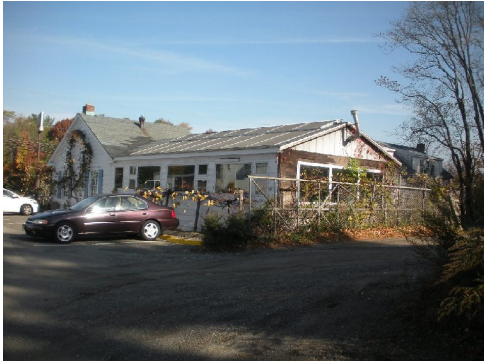
REAR VIEW OF THE FRONT/WEST COMMERCIAL/RETAIL BUILDING
