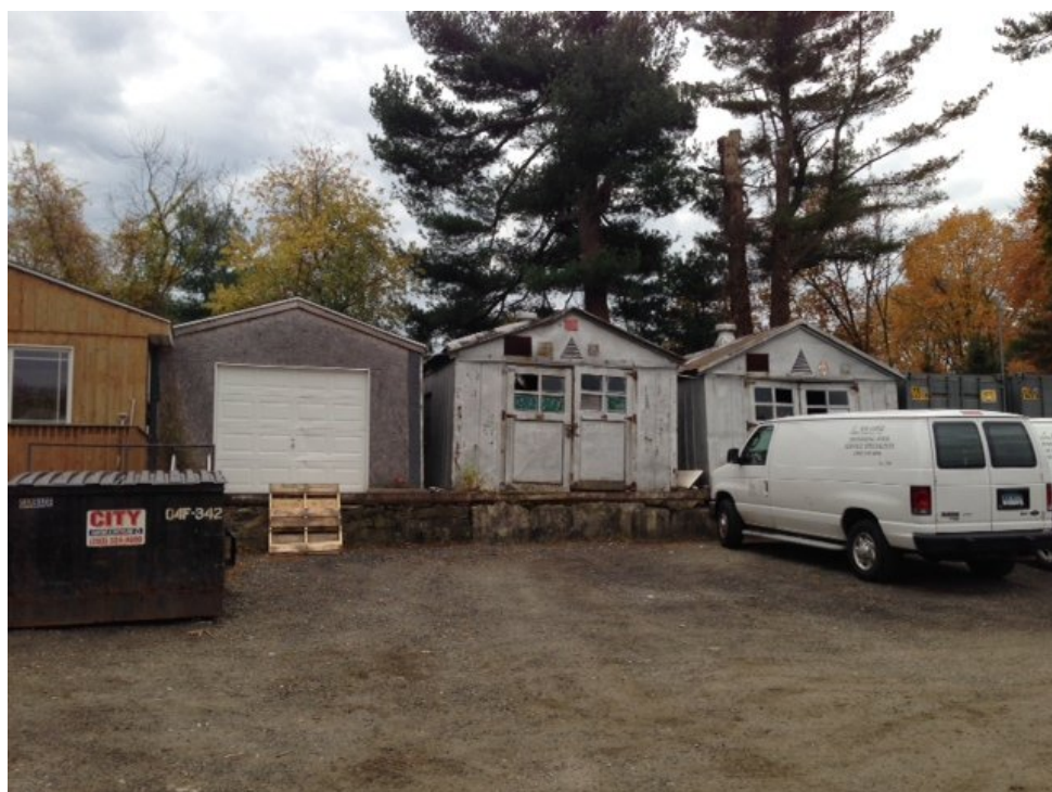
ANCILLARY STORAGE SHEDS AND GRAVEL PARKING AREA
