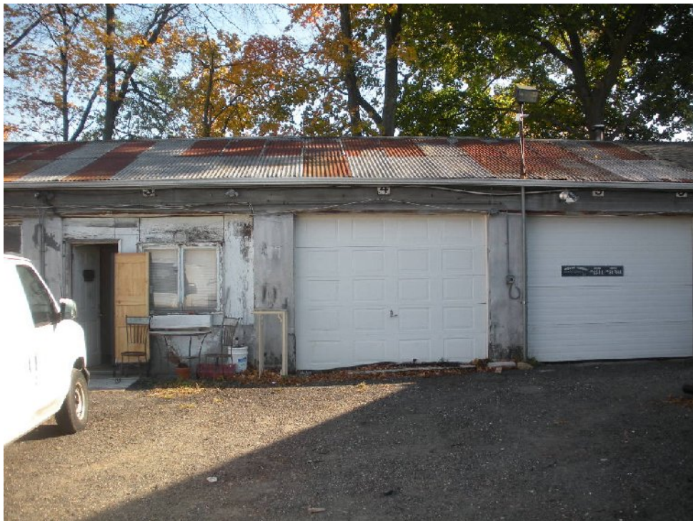
FRONT VIEW OF COMMERCIAL GARAGE/WAREHOUSE BUILDING
