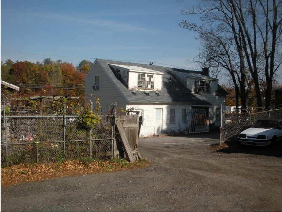
REAR VIEW OF THE FRONT/EAST COMMERCIAL/OFFICE BUILDING
