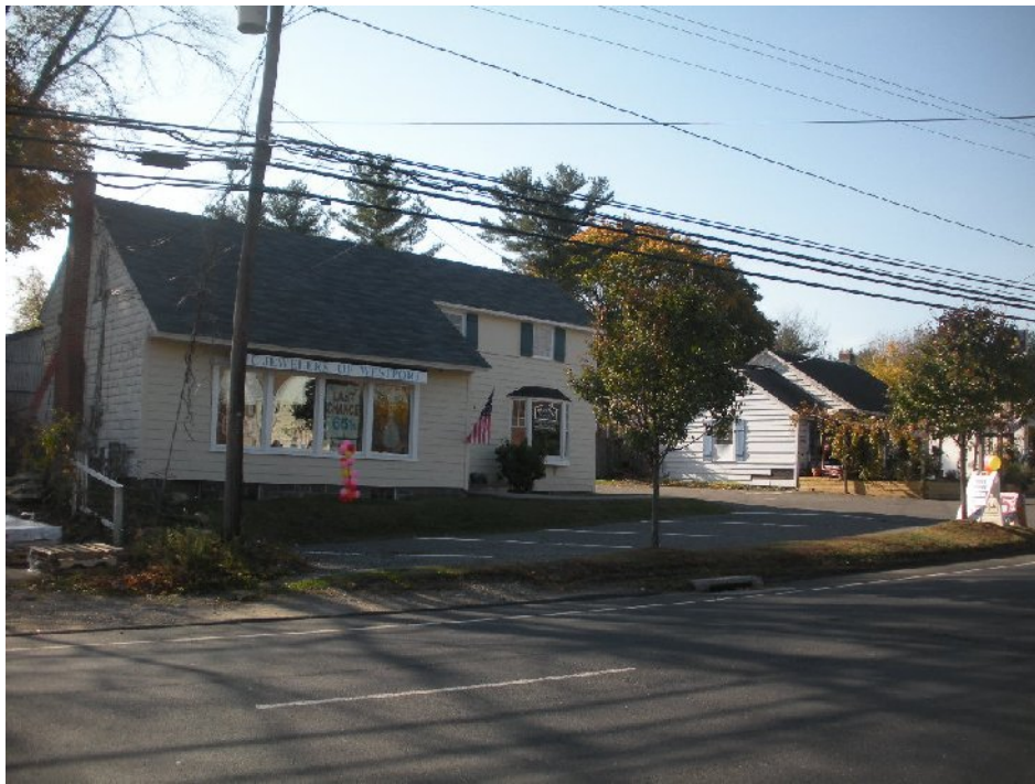
FRONT VIEW – LOOKING SOUTHEAST
