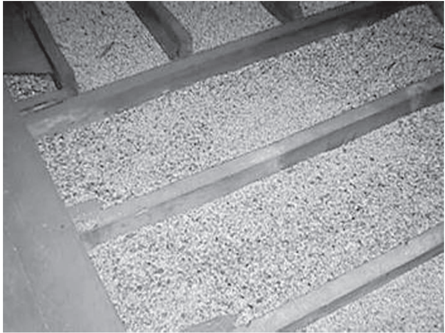
Figure 4: Closeup of Vermiculite Insulation in an Attic
